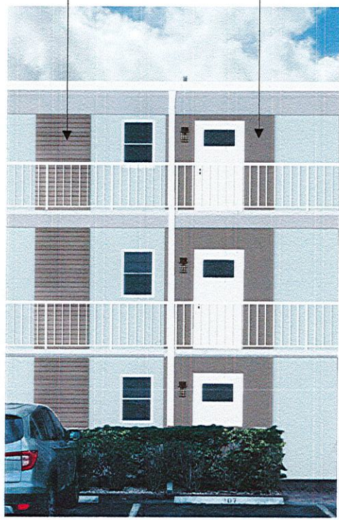
horizontal plank panel to conceal existing door in driftwood
